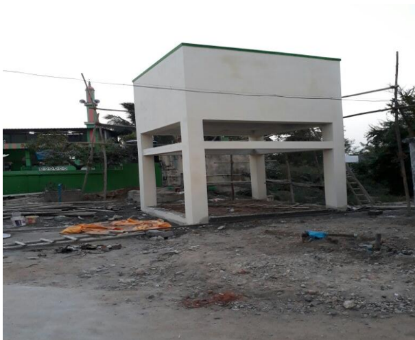
Water tank constructed by Oruma
